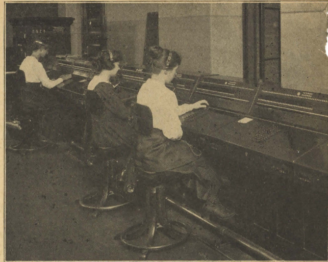
Figure 19. Typical installation of Cordless B positions
