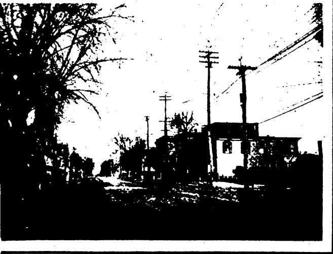
is located about nine miles southeast of Camden. It is a stations. The four views here reproduced show how our construction on the main streets was placed underground. removed with the exception of those owned by the Electric
