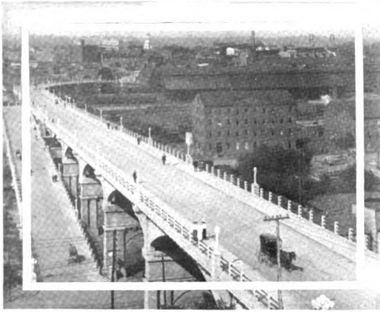
New Concrete Mulberry Street Viaduct, Connecting Business Section of Harrisburg with Residence Section Known as Allison's Hill
