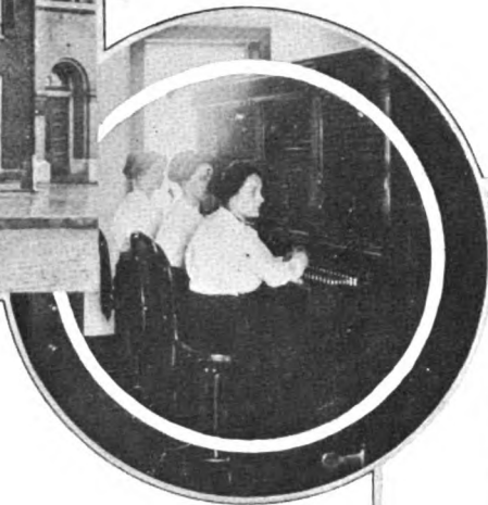
Part of New No. 9 Switchboard— 3 Positions, 200 Local and 30 Rural Lines. (Ultimate 9 Positions, 800 Lines)
