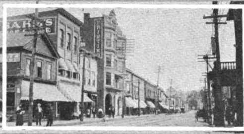
Three Street Scenes and a Large Coal Breaker at Carbondale, Pa.
