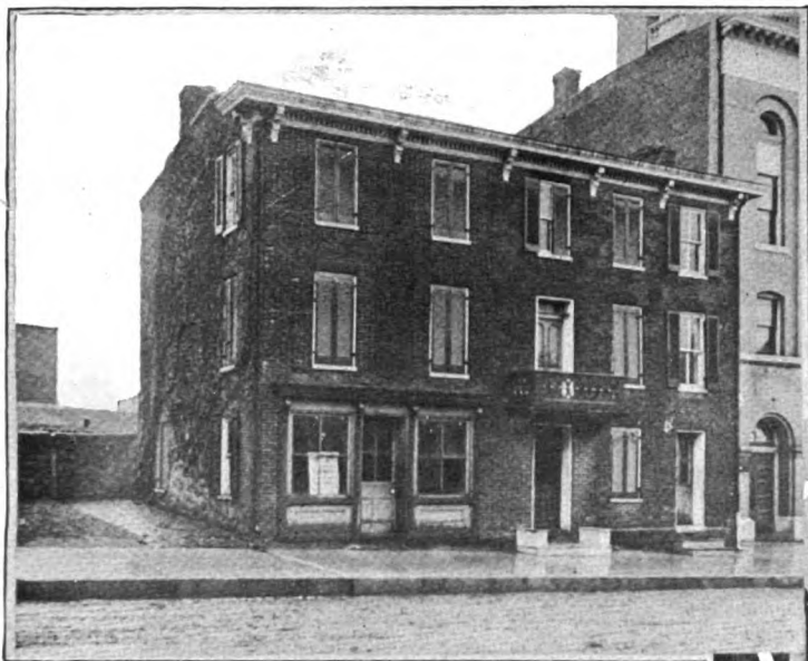
The Westminster, Md., Telephone Building Before and After Alterations were Made. The Colonial Design is Well Preserved
