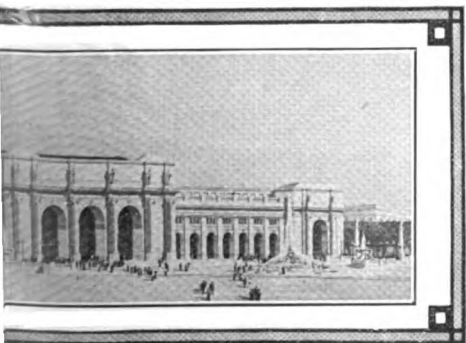
This Building, Completed in 1907, Contains Unusually Elaborate Telephone Equipment
