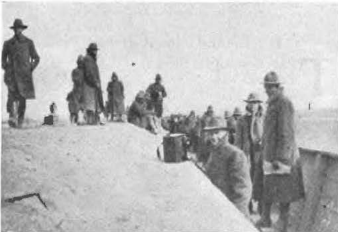
A Western Electric Telephone on the Rifle Range at Camp Logan
