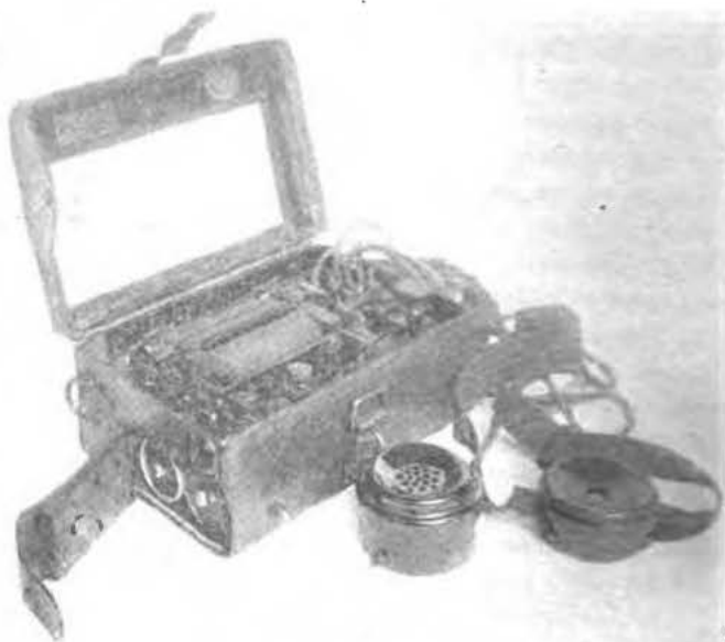
Service Buzzer with case open
