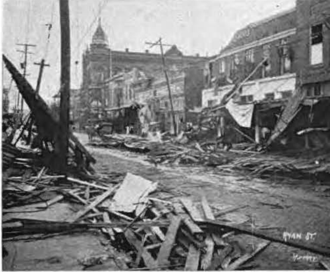
Ryan Street in the heart of Lake Charles. This scene is typical of the destruction caused by the storm
