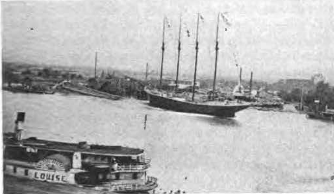
The "Rosalie Hull" leaving the ways and gliding into the Savannah River. This photograph was taken from our Savannah warehouse and, during construction, the "Rosalie Hull" was guarded at night by Western Electric floodlights
