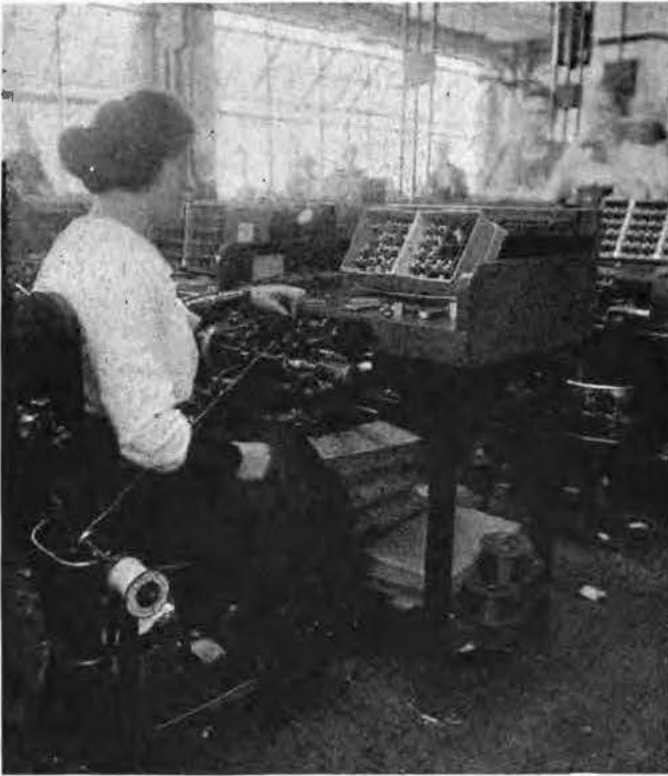
Fig. 8—The Semi-Automatic Coil-Winding Machine
