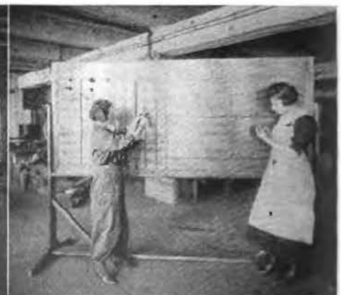
Switchboard Wiring. Miss Bertha Campbell and Miss Violet Price
