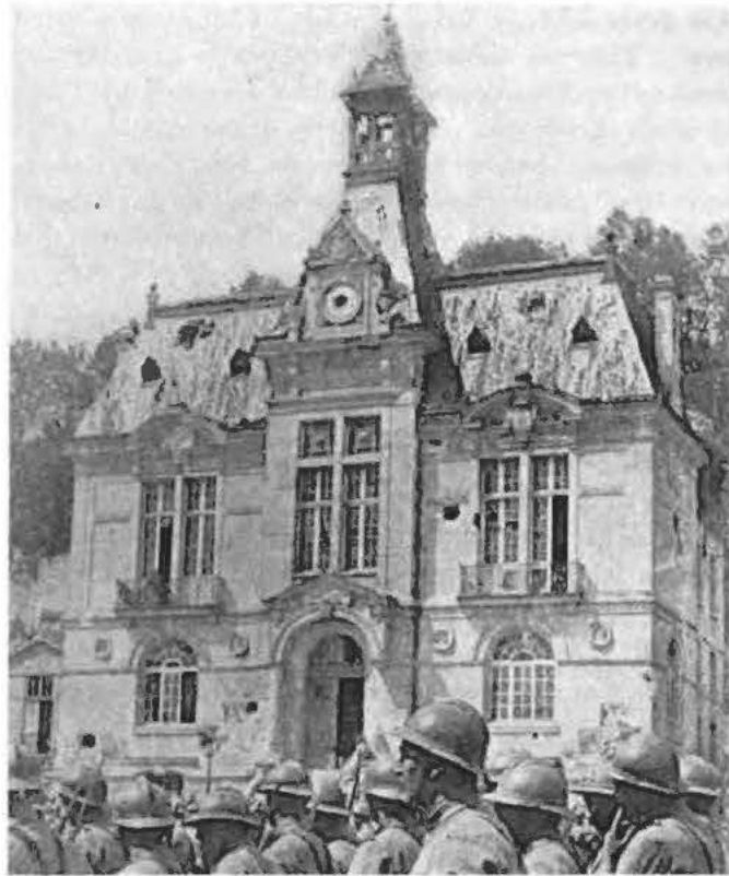
The Hotel de Ville (French for City Hall) in Chateau-Thierry. A German Shell Pierced the Clock Right in the Center
