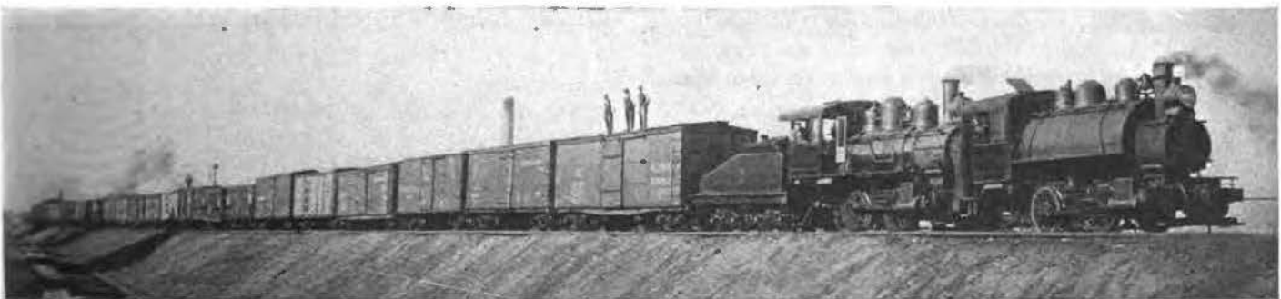
Cars full of cables
