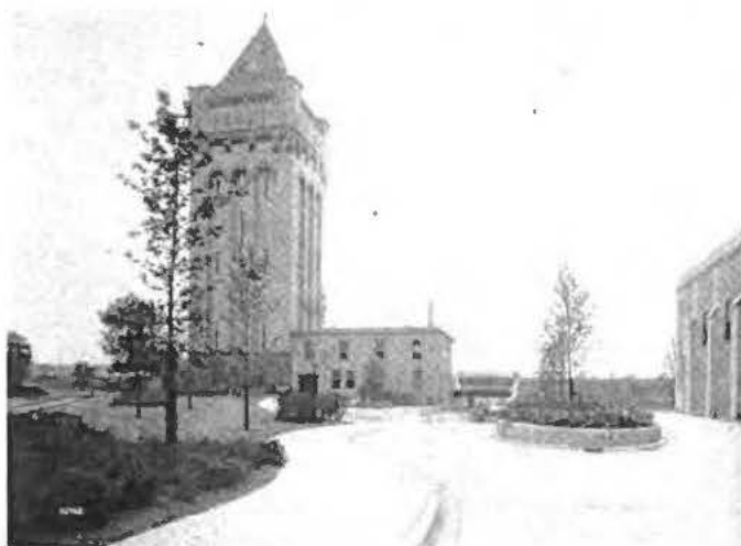
Landscape Work Near the Water Tower
