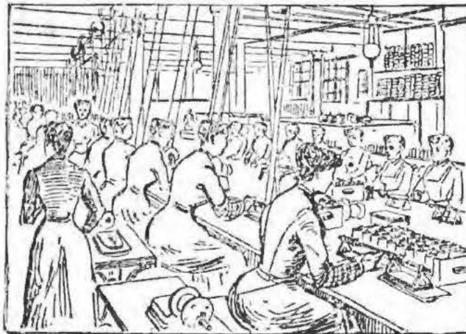
The Insulating Room in the Early Days. From An Old Copy of the Chicago Tribune
