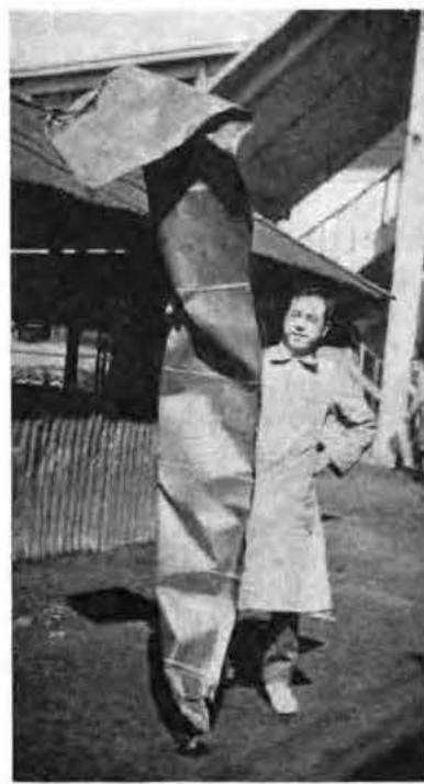
Mr. Hirata Holding a Piece of Copper Sheathing Ripped Off the Roof By the Storm
