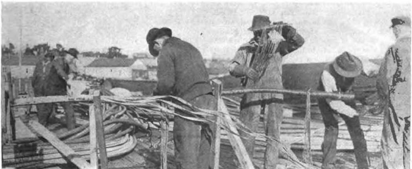
Splicing the Sections and Packing Jute on the Splices
