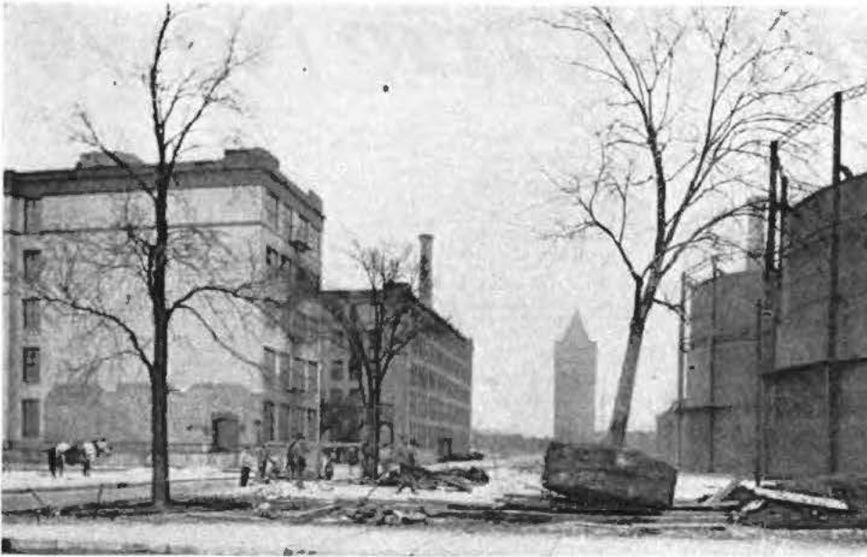
A Grove in the Making. The Transplanting Operation is Completed on the Tree in the Background. The One at the Left is in Place, But the Dirt Has Not Yet Been Filled in Around It. The Tree at the Right is on the Skids Ready to Be Slid Into Place in the Hole Near It
