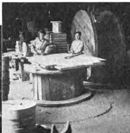
Girls Construct and Repair the Cable Reels
