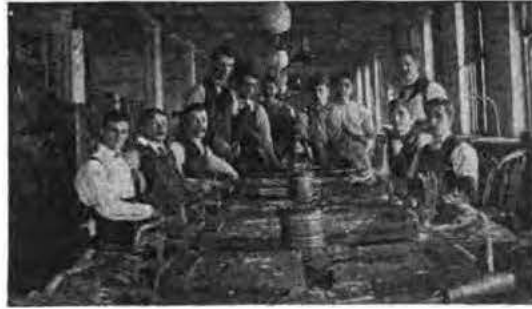
Old Clinton Street Cable Soldering Group
