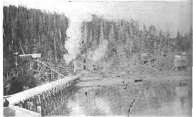
Power house and dock of the Granite gold mine, at Prince William Sound
