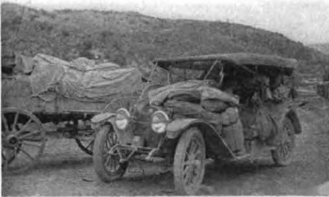
Moving a Construction Camp for 16 Men—In One Day
