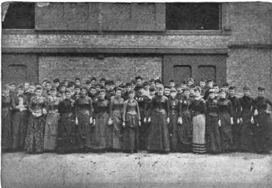
Picture taken in the back yard at Clinton Street in 1886. Girls employed in skeining cotton, manufacturing switchboard, magnet wire, and insulating the textile-covered wire used for pulling into lead pipe, required by early methods of manufacturing lead-covered cable.
