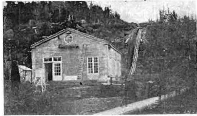
Power House. Citizens Water, Light & Power Company at Ketchikan, Alaska
