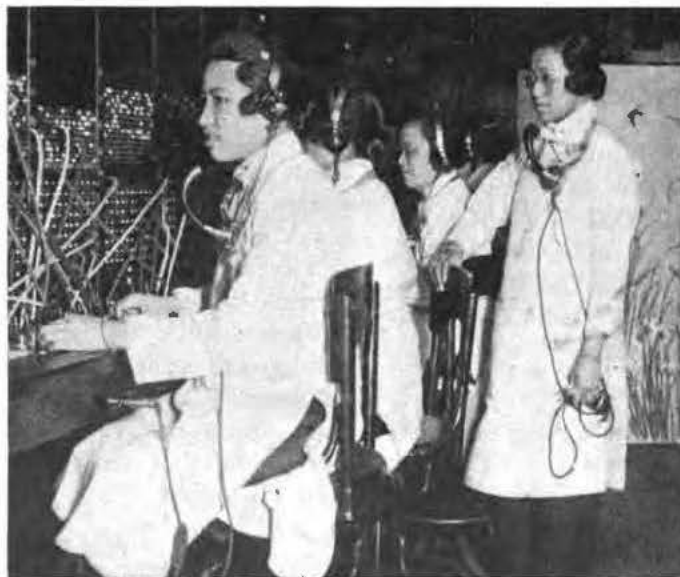
Switchboard, Chinese Telephone Exchange, The Pacific Telephone and Telegraph Company, San Francisco
