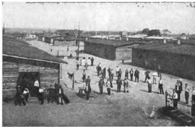
General View in the Prison Camp at Gustrow, Germany
