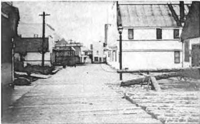
Petersburg. The Western Electric poles in the foreground are for the new municipal electric light system
