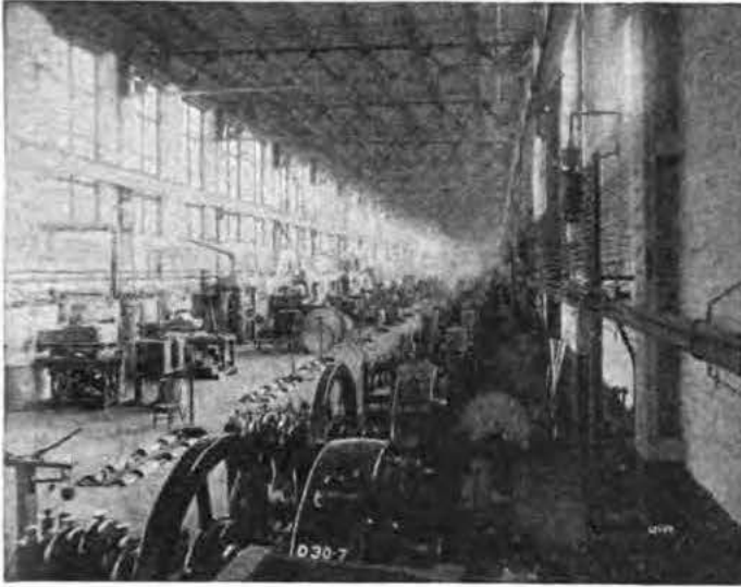
Hawthorne Lead Press Rooms showing, at the right, hydraulic pumps which supply the enormous pressure necessary to force the plastic lead through the die blocks of the presses.
