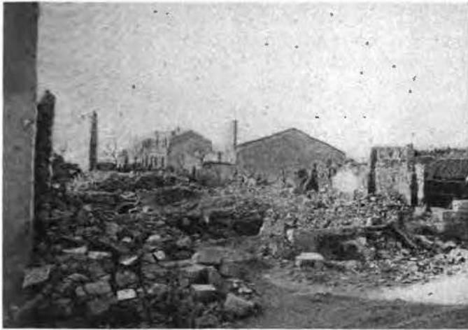
Doesn't Home Look Good Beside This Roofless Billet You Occupied in France?
