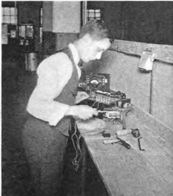
Student Receiving Instruction in Mechanical and Electrical Adjustment of Relays
