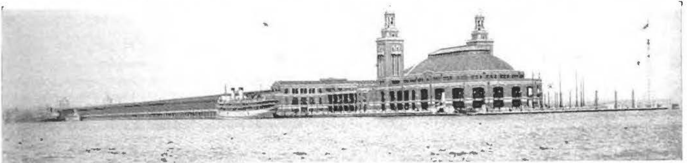
Another View of Chicago's $4,000,000 Pier. It Extends Three-Quarters of a Mile Straight Out Into Lake Michigan. This Will Soon Gleam with Western Electric Sunbeam Mazda Lamps
