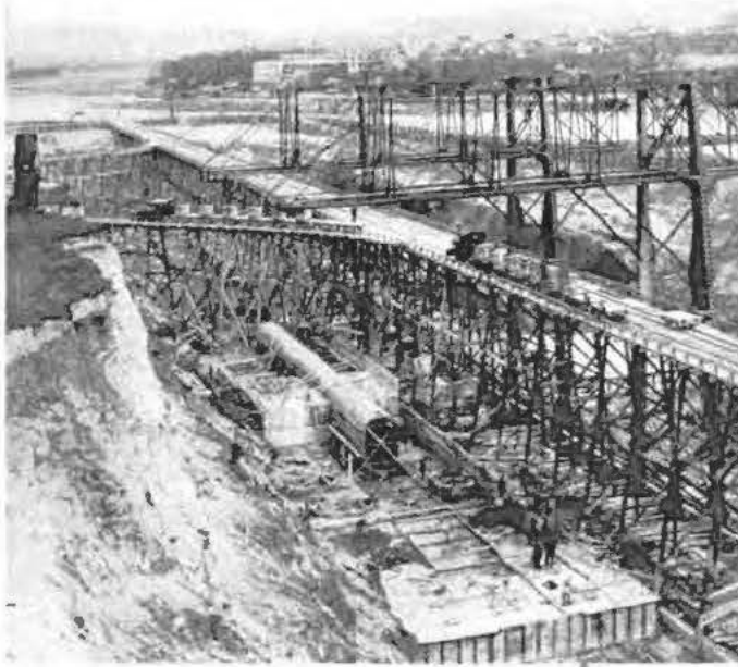
The Immense Size of the Excavation Necessary
