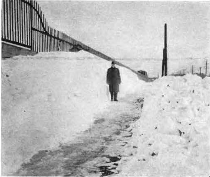
A Trench Through One of the Drifts on Ogden Avenue
