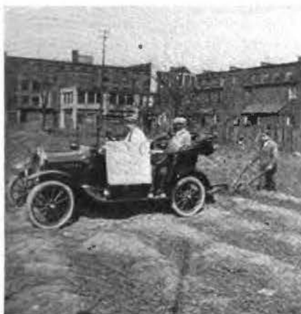
Stores Manager West's Ford Furnishing the Motive Power for Plowing Up the Potato Patch Next to Our Cleveland Telephone Warehouse
