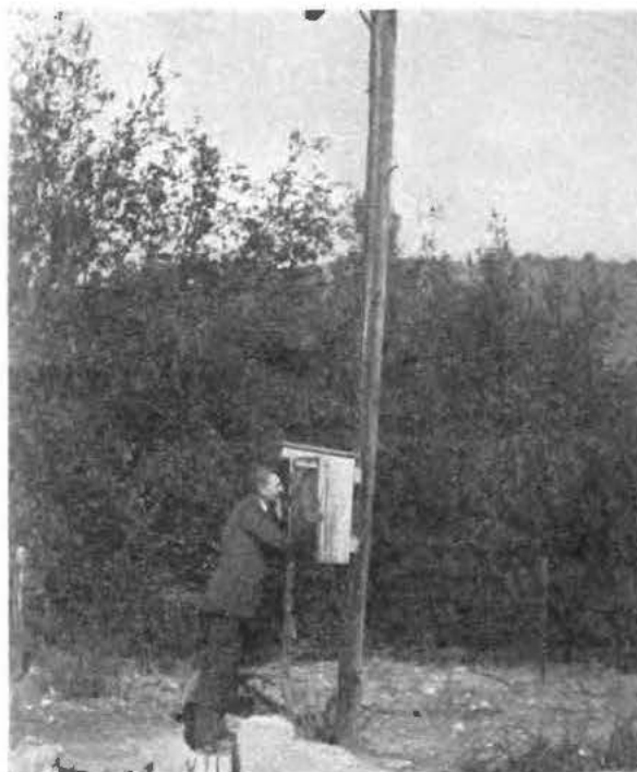
"Is the Track Clear?" W. E. Railway Telephones in South America (Chile)
