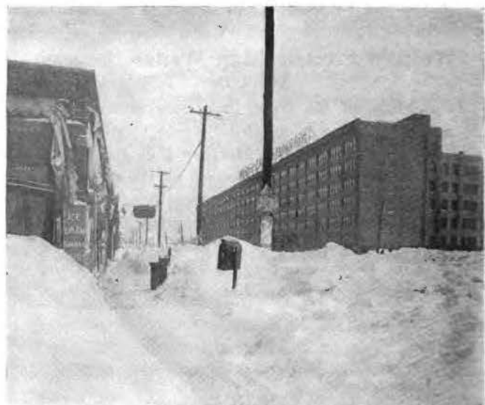
Twenty-second Street looking toward T. A. Building. Somewhere in the drift to the right is a motor truck completely buried.
