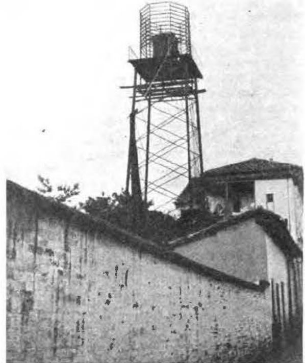
Characteristic Distribution at a Typical Small Telephone Exchange in Brazil
