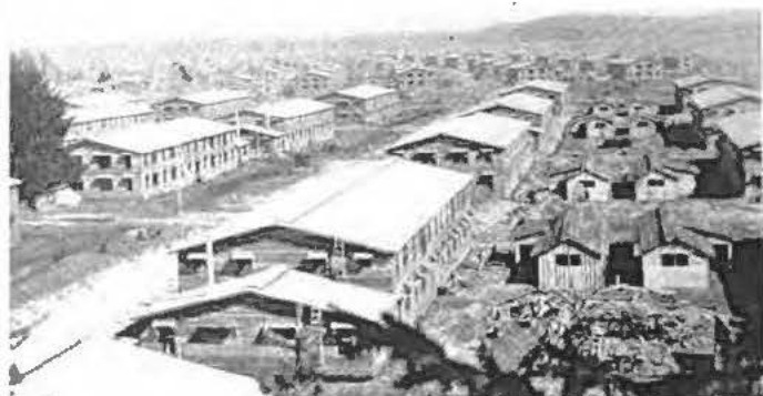
Cantonment at American Lake, Wash., Under Construction
