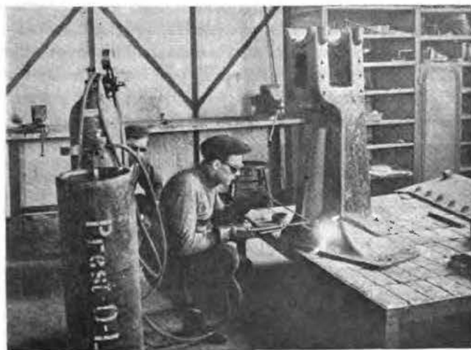
Fig. 2. Soldering the Break With Iron Melted in the Intense Oxy-Acetylene Flame
