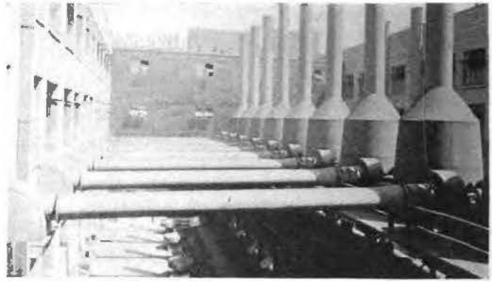
Fig. 3—Cyclones Which Catch the Dust Sucked from the Buffing Machines
