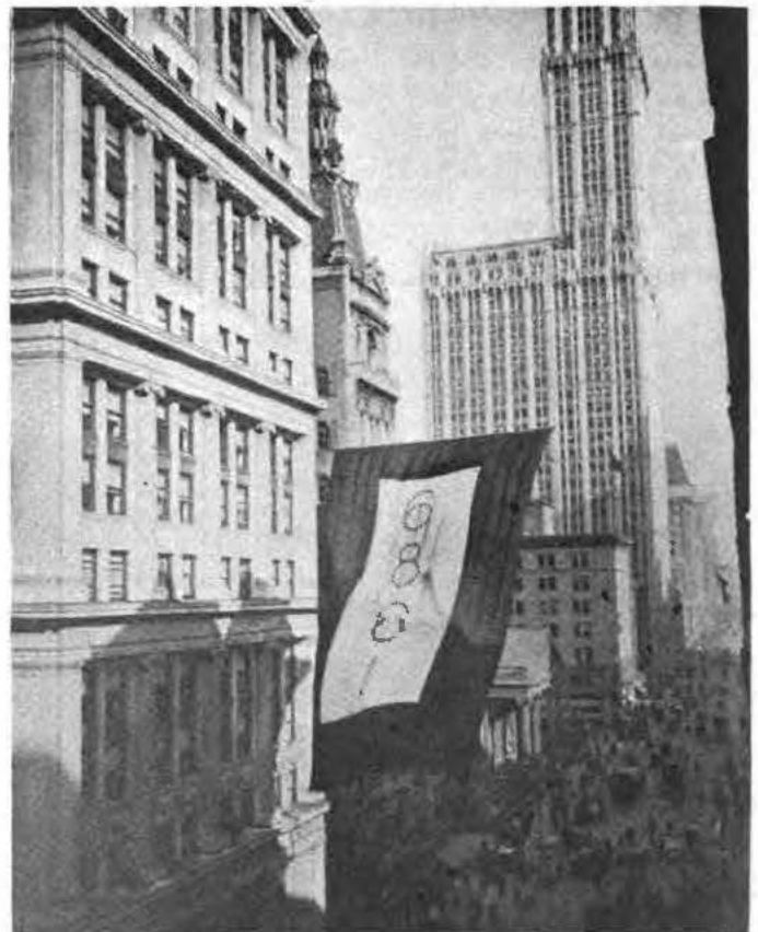
The Service Flag Which Floats Over Broadway in Front of the Telephone and Telegraph Building. The Figures Show the Number of Bell System Employees Who Are in Service, Including Those from the Western Electric Company
