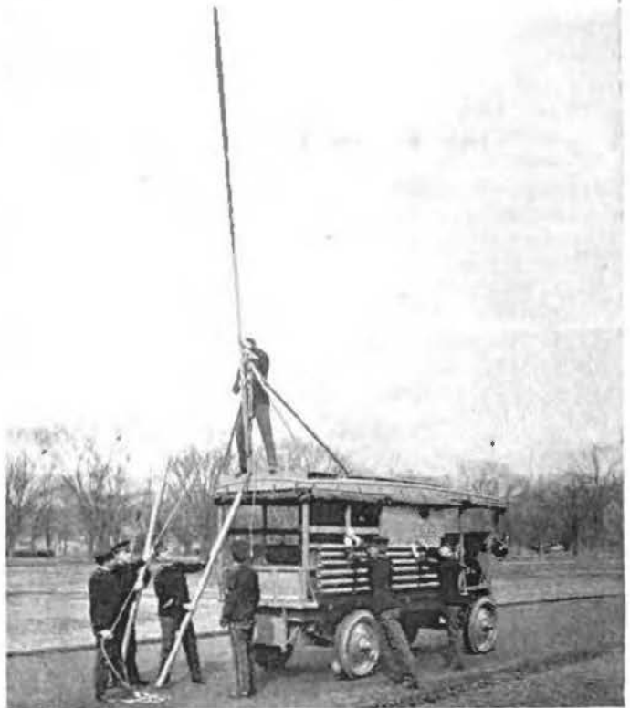
Erecting the Mast for a Tractor Set—Wireless Telegraph
