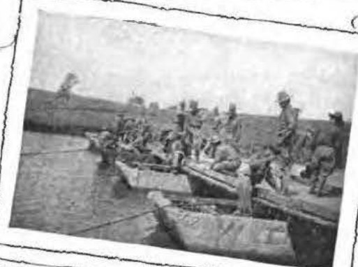
BUILDING A LIGHT PONTOON BRIDGE
