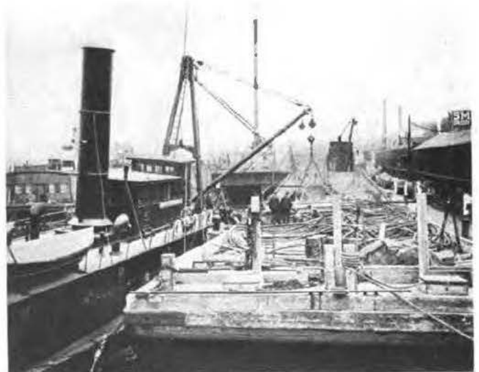
The 16,000-pound Strand Run from Shackle at the Top of the Sling and Fastened to Cable to Ease the Strain Near the Loading Pot When Lowered Into the Water
