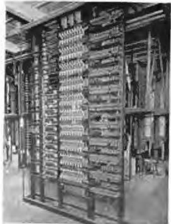
Fig. 8. Sender equipment in process of assembly at factory
