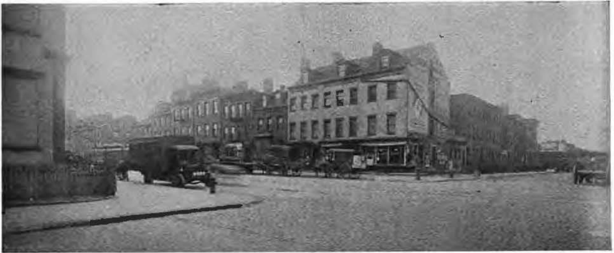
An excellent view of the block which will be occupied by the new 395 Hudson Street building. The corner gable house in the foreground is more than 100 years old. It is being destroyed
