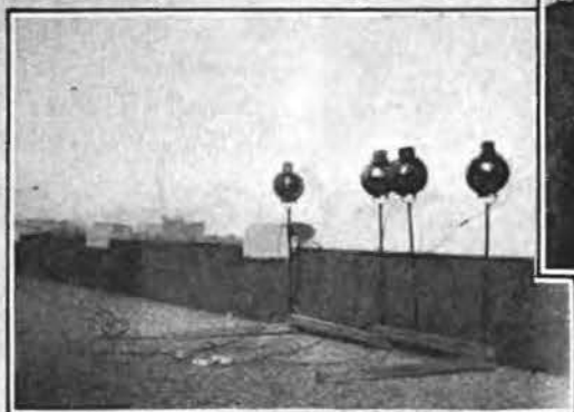
Four 1,000 watt Flood Lights atop the Boston house, helping light up the city harbor.
