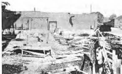
This picture shows how the new building will fit in with the present Emeryville plant
