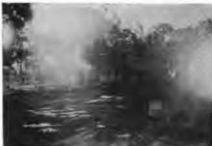
This photograph, though somewhat blurred by the falling eucalyptus tree, is most interesting in that it shows how these evergreens at Emeryville had to be felled to make room for building
