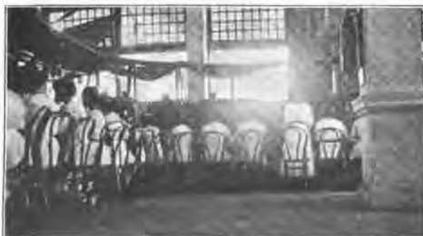
Singapore Exchange before and after—Note absence of supporting racks for cable, which is secured by rope. Even with this poor equipment fairly satisfactory service was given during the years following the fire, before the new board was installed
