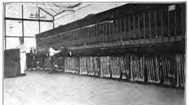
Singapore Exchange before and after—Note absence of supporting racks for cable, which is secured by rope. Even with this poor equipment fairly satisfactory service was given during the years following the fire, before the new board was installed
