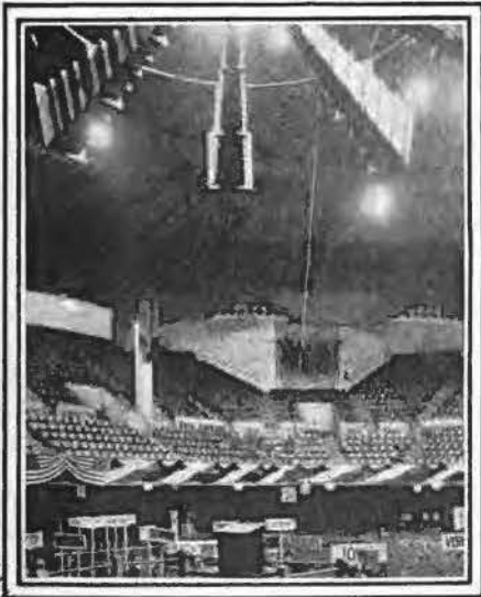
VIEW LOOKING OUT OVER THE DELEGATES SECTIONS PAST THE SPEAKERS TABLE. THE THREE RECTANGULAR BOXES CONTAIN THE TRANSMITTERS USED TO COLLECT ENERGY FROM THE SPEAKERS VOICE. THIS ENERGY WHEN SUFFICIENTLY STRENGTHENED BY THE AMPLIFIER WAS EXPENDED IN THE LOUD SPEAKING RECEIVERS SHOWN ABOVE.
