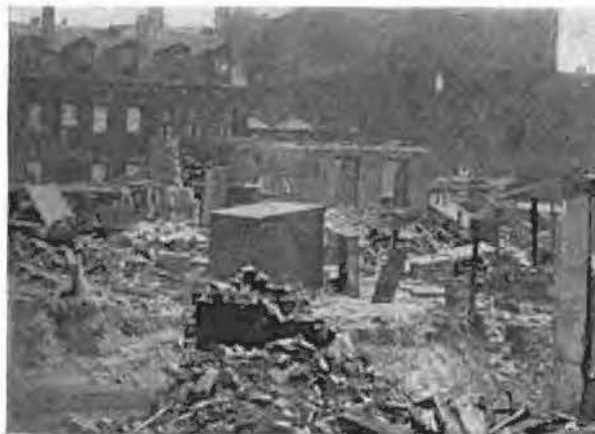
An entire block of old houses is being demolished
