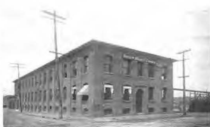
This is the New Home of the Providence Western Electric Fan
