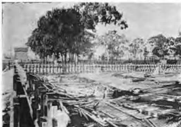
An excellent view of the Emeryville construction under way
