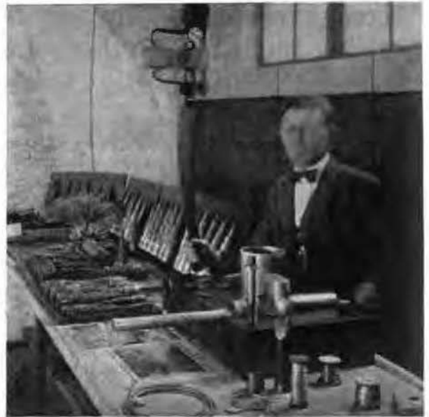
Big lead press dies, showing how the sheath is formed around the cable. The murderous looking cutlass is an innocent knife used by the operators to cut the end of the sheath after the cable is completed
