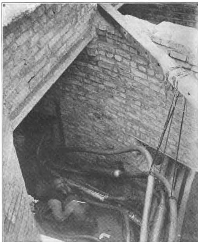
FIGURE 3.—TEMPORARY SUSPENSION OF CABLE
