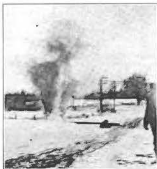
BLOWING POLE HOLES WITH DYNAMITE.
