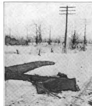
POLE AND CABLE BOX DOWN. Part of a break of thirty-nine poles six miles northwest of Libertyville, Ill.
