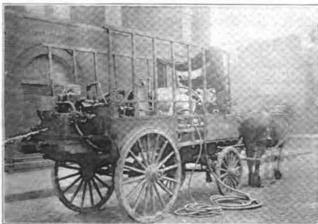
COMPRESSED AIR MACHINE FOR DRYING CABLES.
