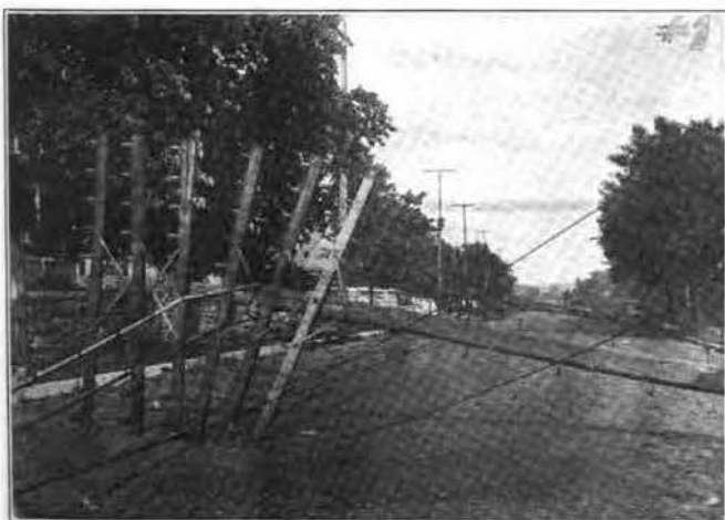
TELEPHONE LINE AFTER ALTON FLOOD.
