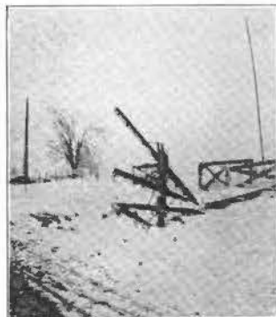
NEAR LIBERTYVILLE, ILL. Part of a break of eighty poles. Many toll leads looked like this.
