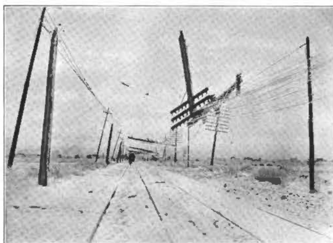
RAVAGES OF ILLINOIS SLEET STORM. Tangle of wires and broken poles in Kedzie avenue, Chicago.
