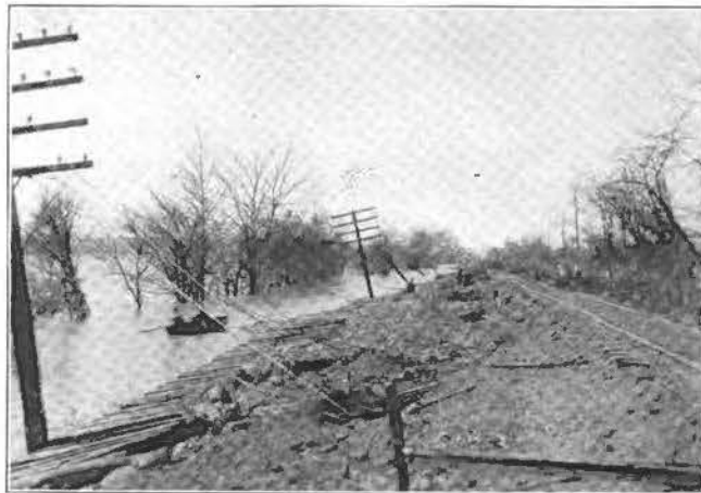
LOUISVILLE-BLOOMINGTON TOLL LINE NEAR TERRE HAUTE. Showing where twisted pair cable was carried under Big Four tracks to make connection with Central Union wires on the right. Twisted pair was strung on Western Union poles for about a mile. Western Union poles standing on the left.
