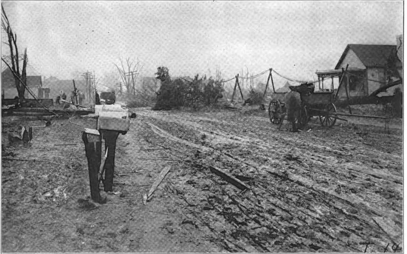
7. 19 AFTER THE CYCLONE AT TERRE HAUTE, IND. Showing twisted pair wire hung on crossed timbers to keep toll communication open.
