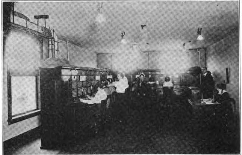
NEW SWITCHBOARD, MONROE, MICH.
