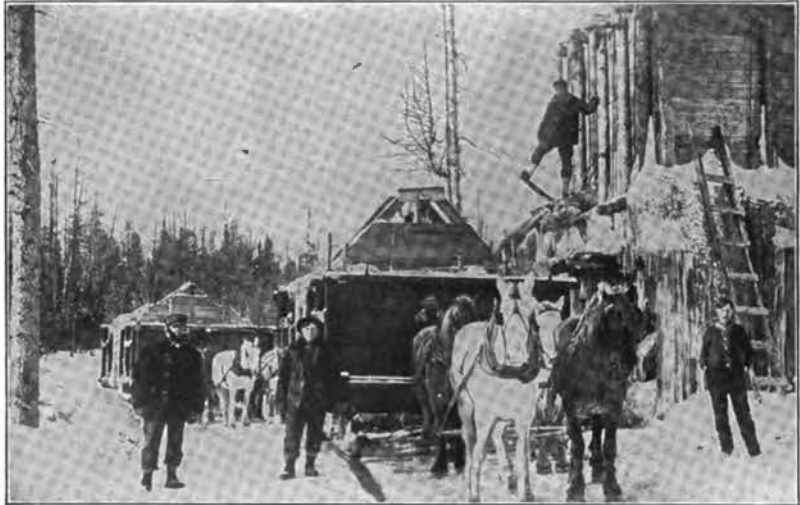
SUPPLY TANK AND SPRINKLERS FOR MAKING ICE ROADS.
