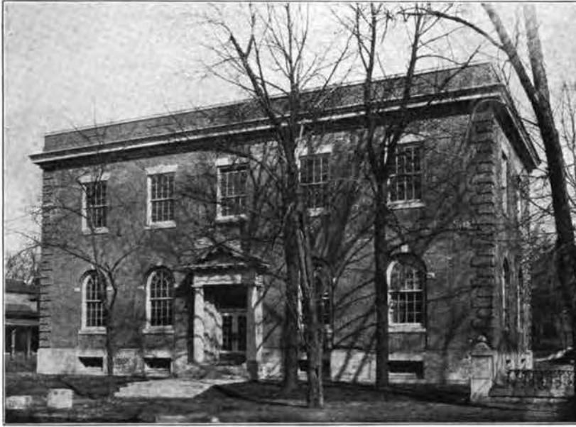
NEW EXCHANGE BUILDING OF THE CENTRAL UNION TELEPHONE COMPANY AT ROCK ISLAND, ILL.
