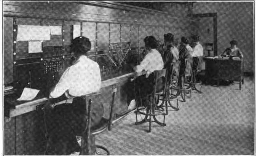
SWITCHBOARD AT MICHIGAN CENTRAL DEPOT, DETROIT.
