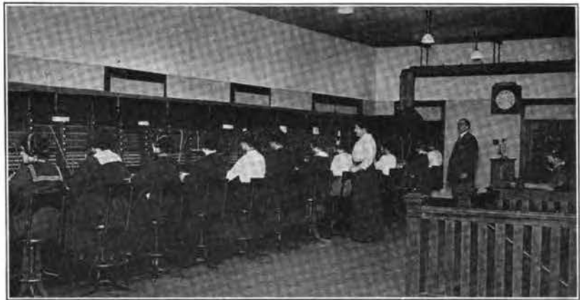
SWITCHBOARD AFTER CUT'OVER AT MT. CLEMENS, MICH.
