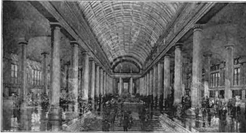
BANKING FLOOR, NEW CONTINENTAL AND COMMERCIAL BANK BUILDING, CHICAGO.
