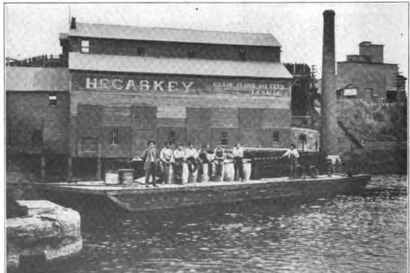
GANG AND CANAL BARGE LOADED WITH TELEPHONE SUPPLIES.
