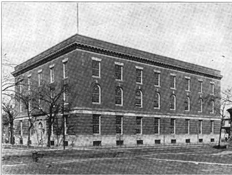
NEW STEWART OFFICE BUILDING, CHICAGO.
