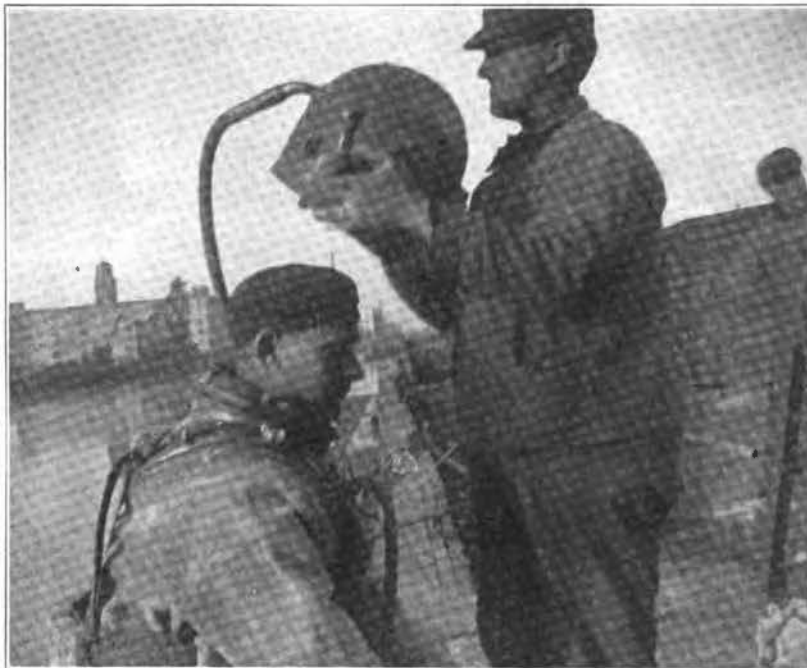
DIVER PREPARING TO ENTER CHICAGO RIVER TO INSPECT PIPES.
