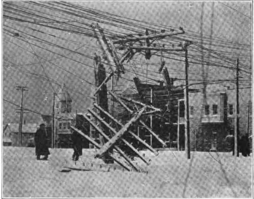
WIRE CONDITIONS AFTER CLEVELAND STORM.
