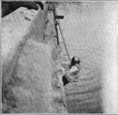
DIVER ENTERING RIVER TO FIX CHAINS TO CABLE REEL.
