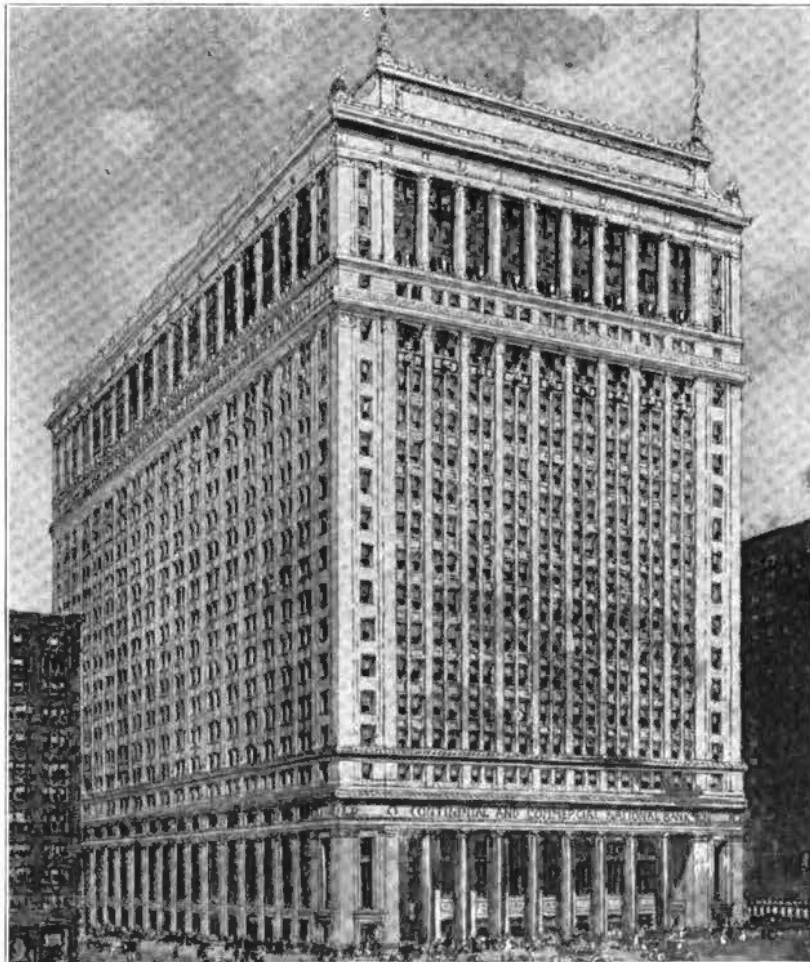
NEW CONTINENTAL AND COMMERCIAL NATIONAL BANK BUILDING, CHICAGO.
