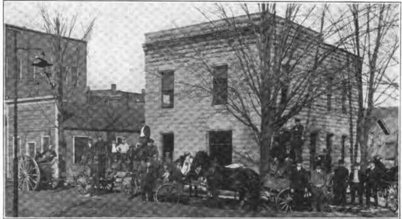
TELEPHONE BUILDING, LAPEER, MICH. Picture Shows Plant Force Which Recently Finished the Lapeer Alterations.
