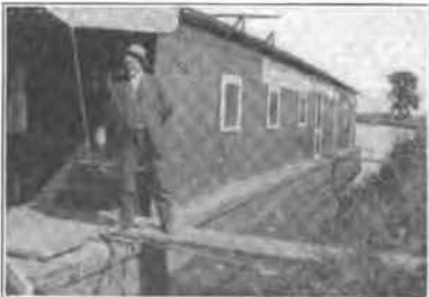
FOREMAN MERRILL IN CHARGE OF TELEPHONE GANG ON ILLINOIS MICHIGAN CANAL.
