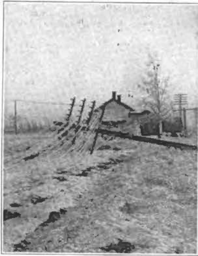
LINE OF EATON, OHIO, TELEPHONE COMPANY AFTER FEBRUARY SLEET STORM.
