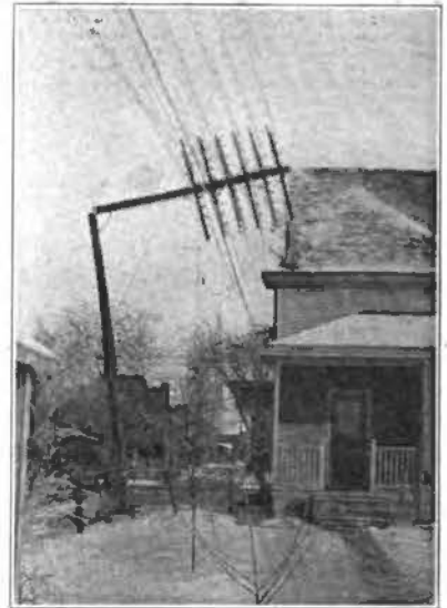
LINE OF EATON, OHIO, TELEPHONE COMPANY, AFTER FEBRUARY SLEET STORM.
