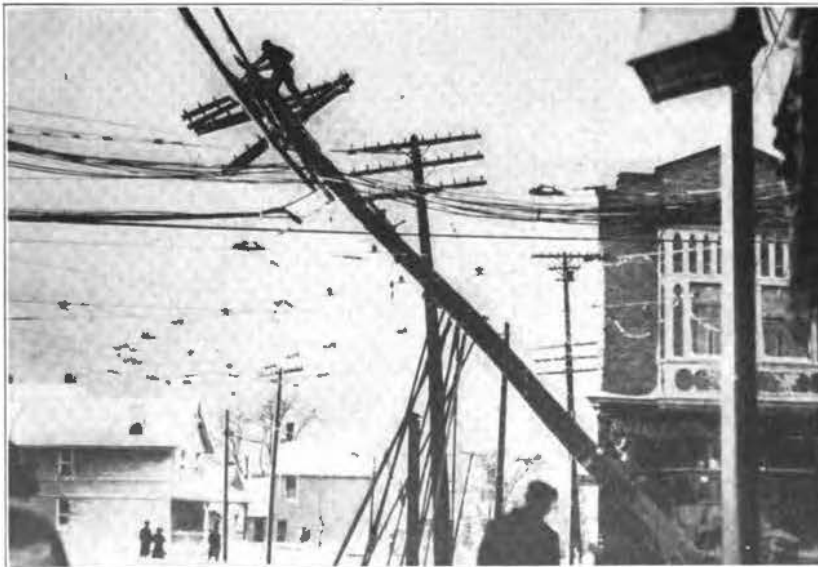
WIRE CONDITIONS IN CLEVELAND AFTER STORM. A Difficult Situation to Clear.
