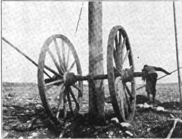
"THE BULL," A HOME-MADE DEVICE FOR MOVING POLES. This picture shows how the chain is fastened to the pole and then wound around the iron-pipe axle.
