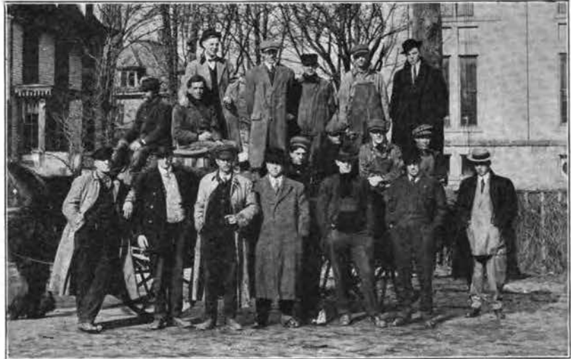
CONSTRUCTION CREW WHICH REBUILT MONROE EXCHANGE.
