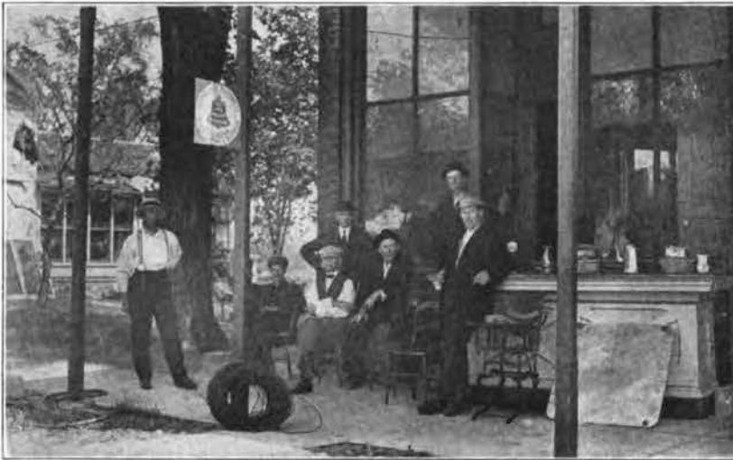
TEMPORARY OFFICE AT BROOKLYN, MICH. Installed After Fire Described on Page Five.
