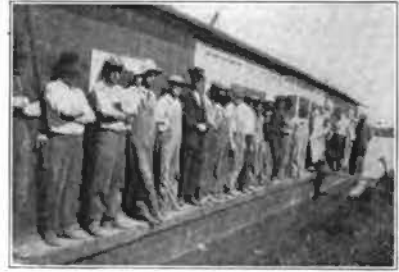
TELEPHONE GANG READY TO START ON ILLINOIS-MICHIGAN CANAL.
