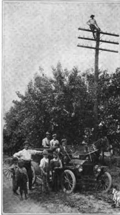
TREE TRIMMING ON TOLL CIRCUITS, GRAND LEDGE, MICH.
