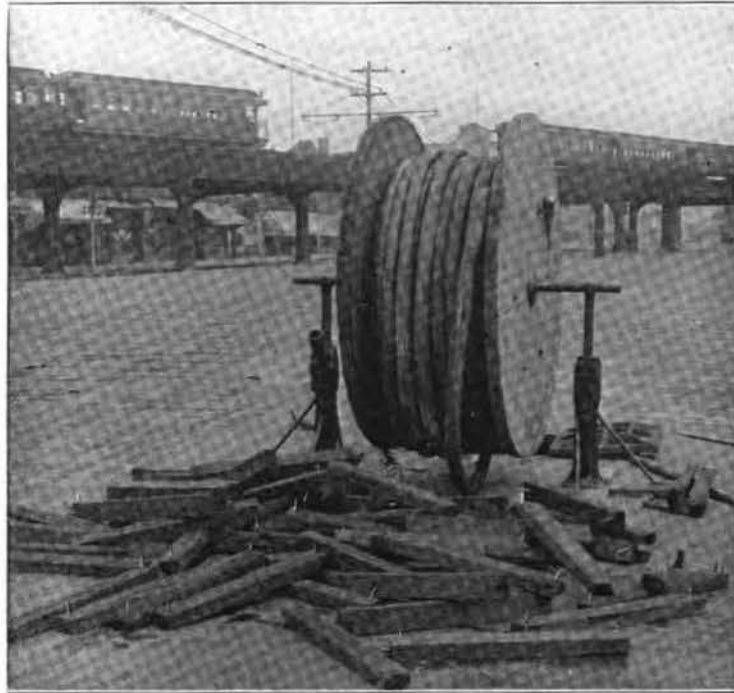
A DANGEROUS SITUATION.
