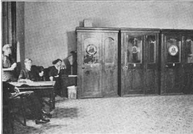
PAY-STATION EQUIPMENT, STATE CAPITOL, LANSING. Operators May Bonesteel and Nan Calvary and House Page McGill are shown.
