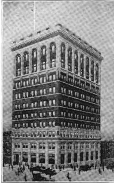
TELEPHONE BUILDING, CINCINNATI.
