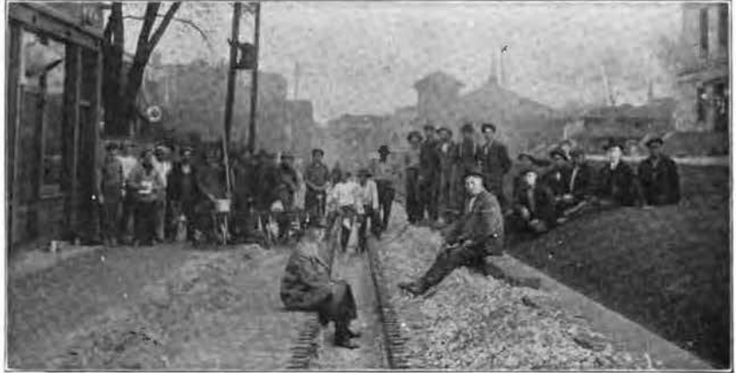
UNDERGROUND WORK IN PROGRESS AT MICHIGAN CITY, IND.
