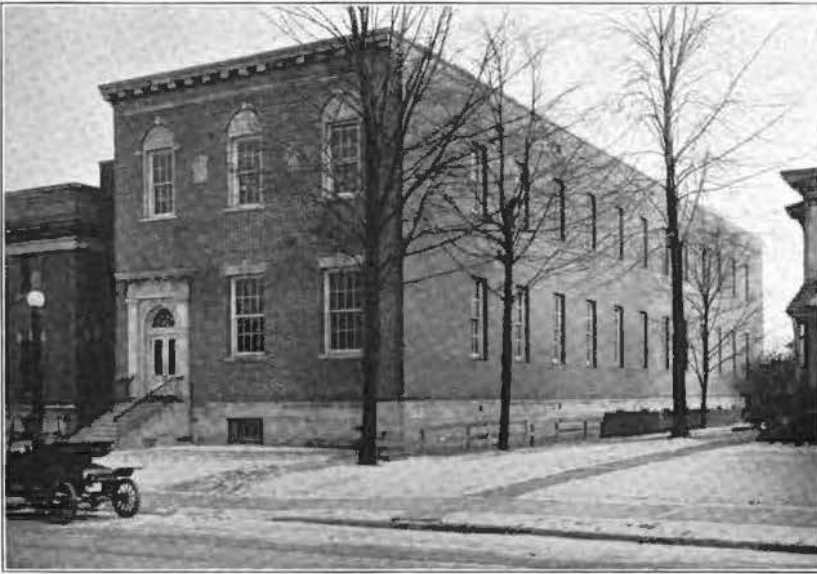
NEW GARFIELD BUILDING, CLEVELAND.
