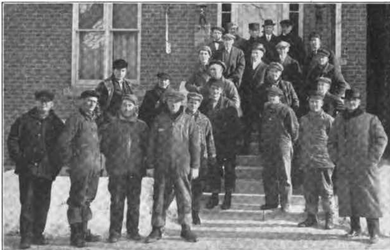
CONSTRUCTION CREW ON ESTIMATE WORK, AND WIRE CHIEF'S FORCE, LINCOLN EXCHANGE, MILWAUKEE.
