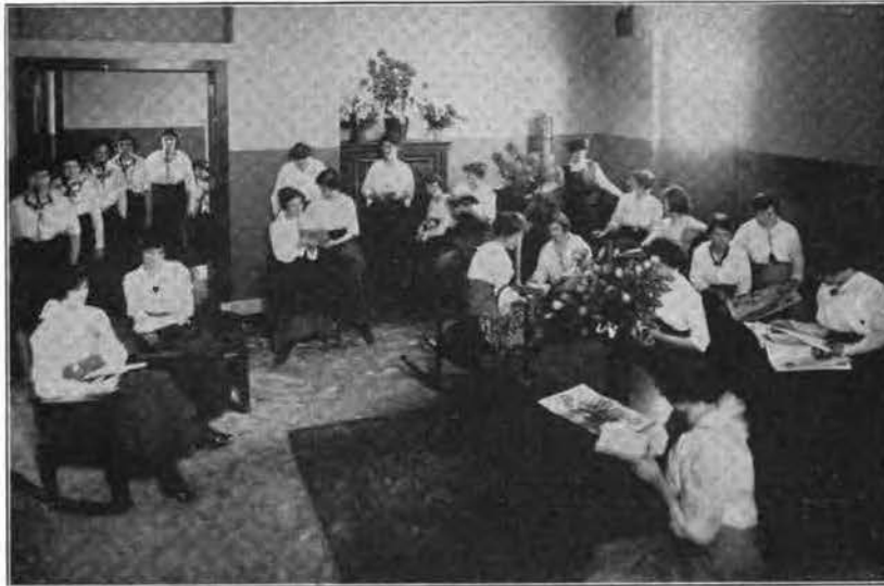
OPERATORS' REST ROOM, GARFIELD OFFICE, CLEVELAND.
