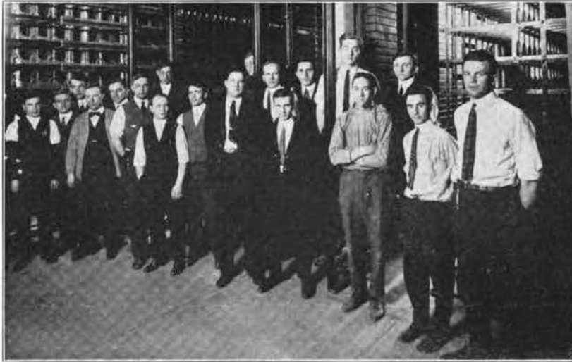
CUT-OVER FORCE IN GARFIELD TERMINAL ROOM, CLEVELAND.
