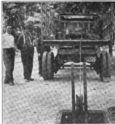
CABLE PULLING TRUCK.
