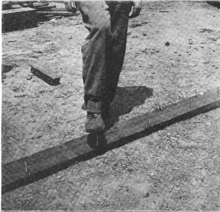
THIS IS ONLY A PIECE OF BOARD WITH NAILS IN IT. But similar pieces have been the cause of a large number of accidents.
