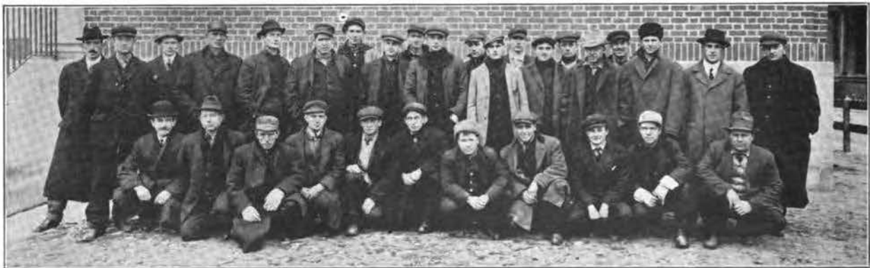
CABLE MEN WHO WORKED ON GARFIELD CUT-OVER.
