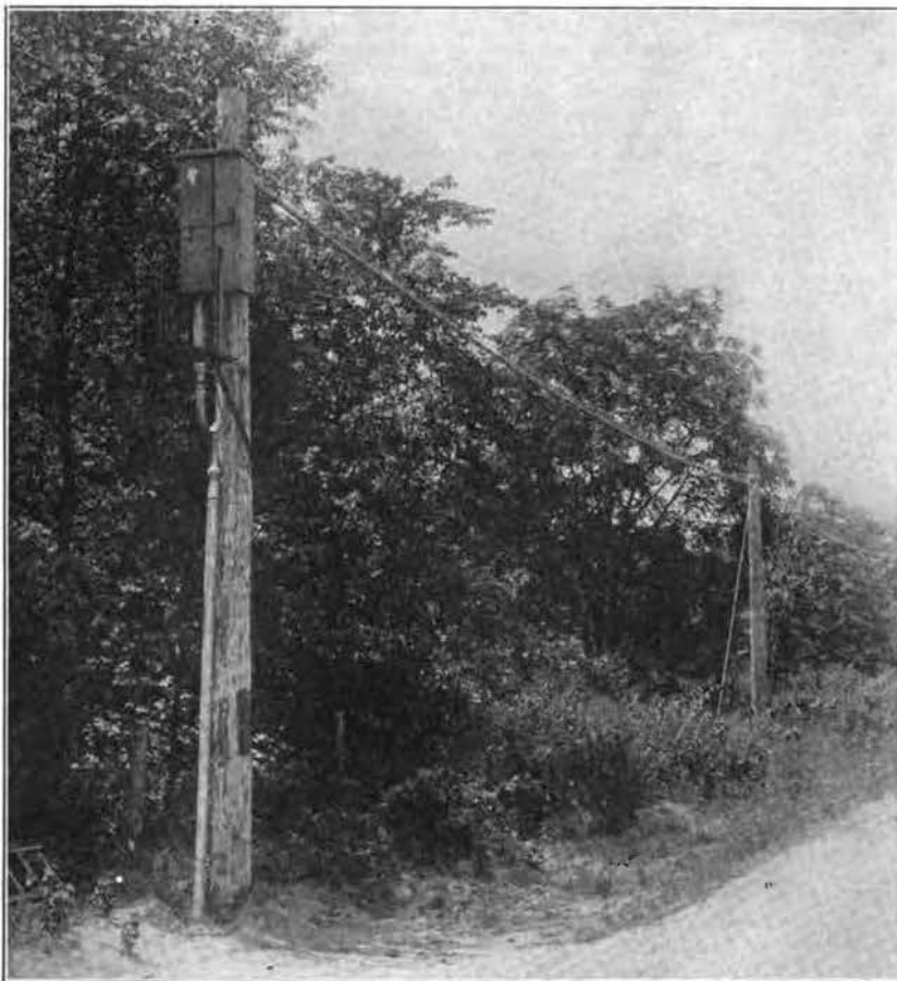
JUNCTION OF NEW AERIAL TOLL CABLE WITH PRESENT CHICAGO-MILWAUKEE UNDERGROUND LINE.
