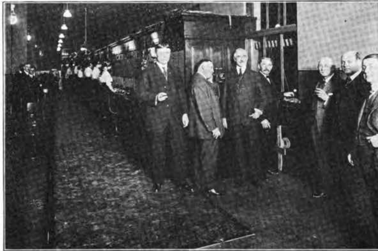
OAK PARK VILLAGE OFFICIALS AND TELEPHONE OFFICIALS AT OAK PARK CUT-OVER.
