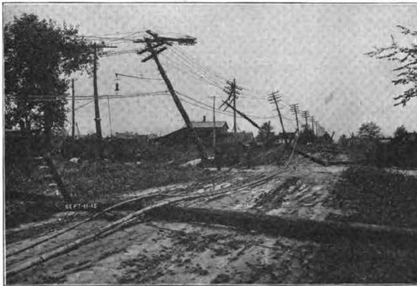
WRECK OF POLE LINES ON KERCHEVAL AVENUE, DETROIT.
