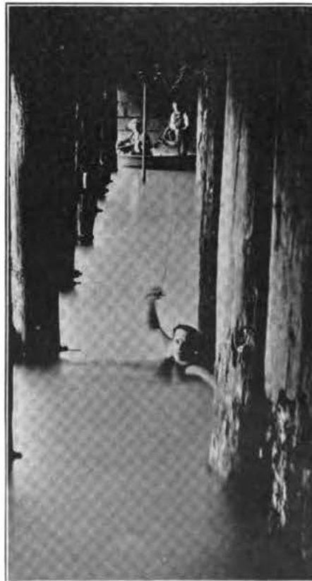
INSTALLER CARNEY CARRYING LINE UNDER LIFE SAVING STATION.
