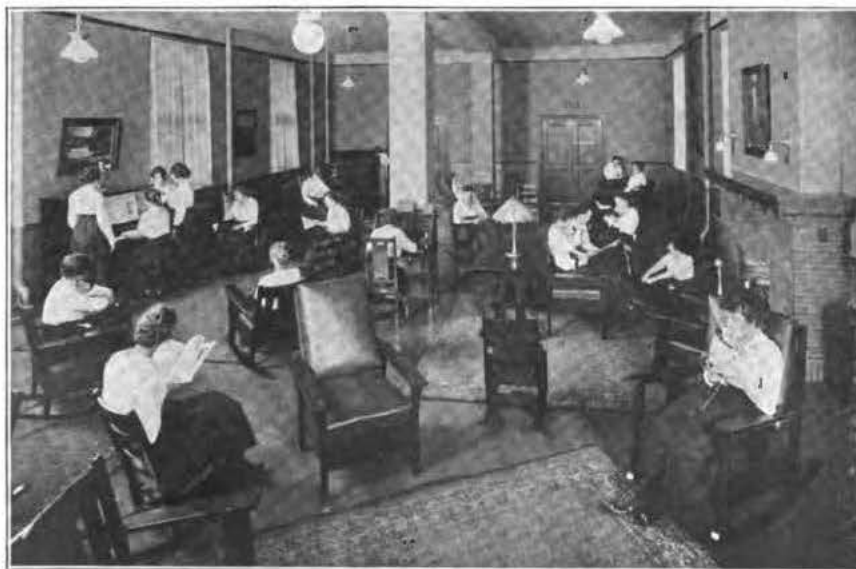
OPERATORS' REST ROOM, NEW HYDE PARK OFFICE.
