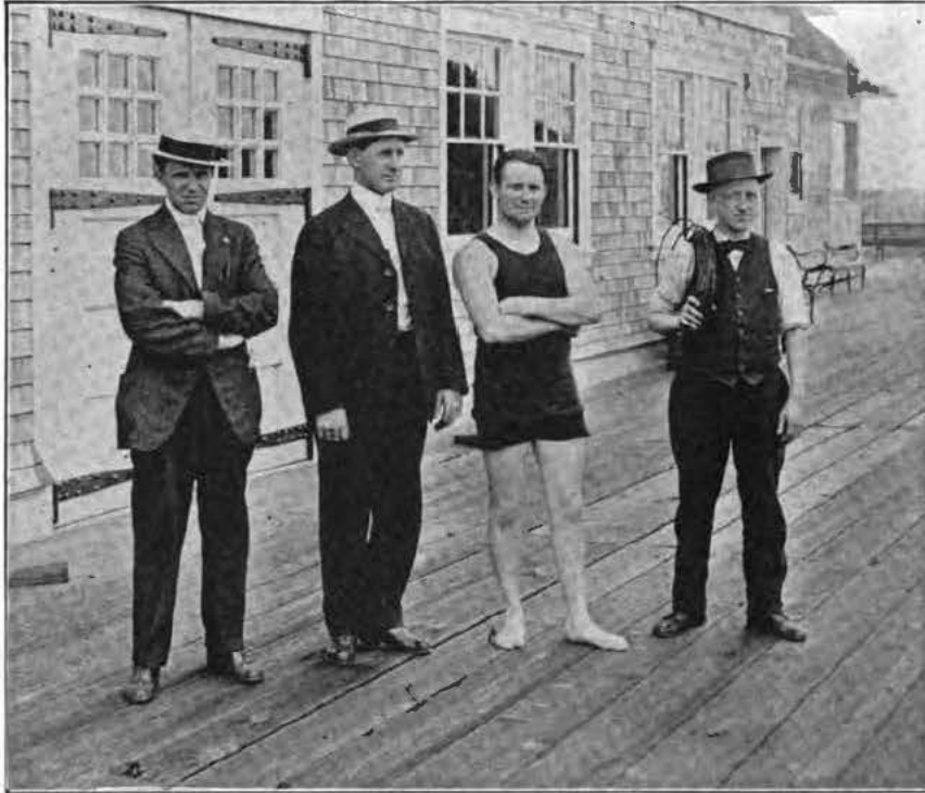
INSTALLER CARNEY (IN BATHING SUIT) AND CHICAGO PLANT MEN READY TO INSTALL EXTENSION SERVICE AT LIFE SAVING STATION.
