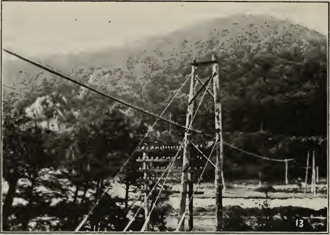
Fig. 9—Cable Crossing at Juniata River
