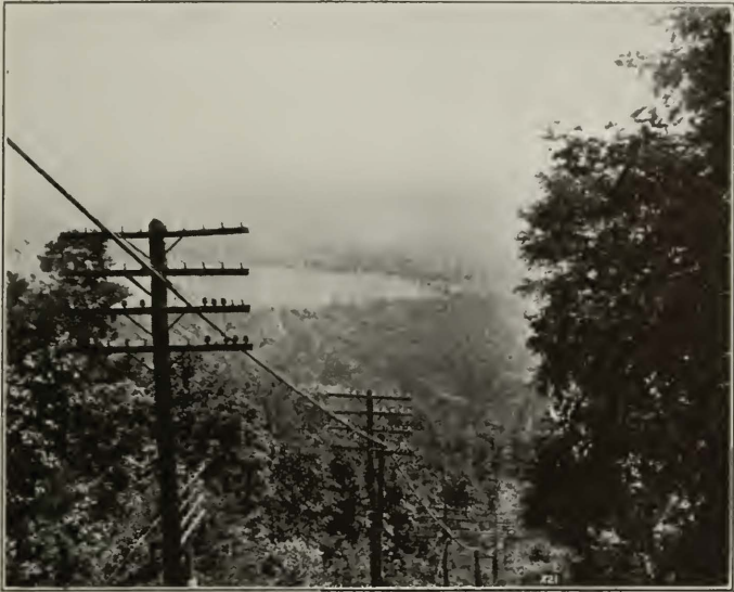
Fig. 8—Cable Line Across Valley at Grand View
