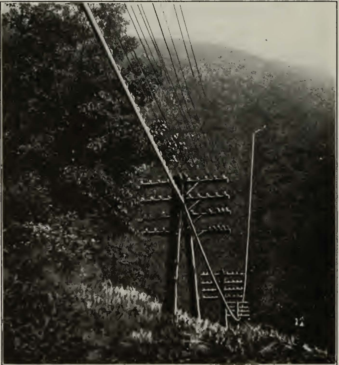
Fig. 10—Cable Line on Steep Slopes
