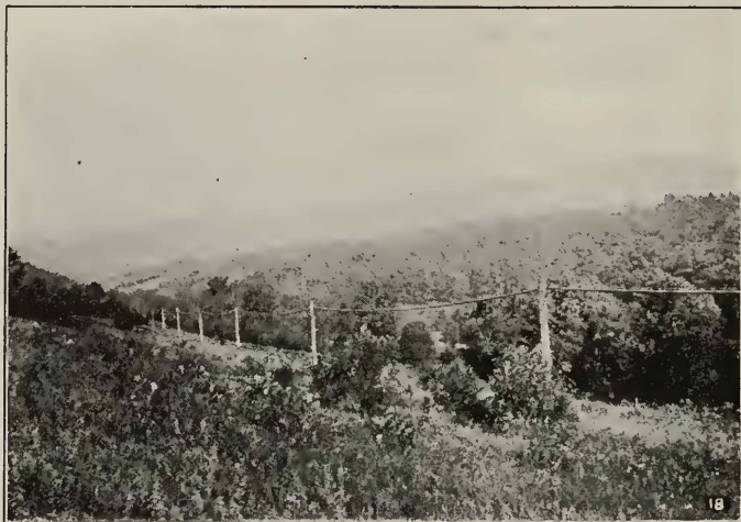
Fig. 5—General View of Pole Line Carrying Aerial Cable
