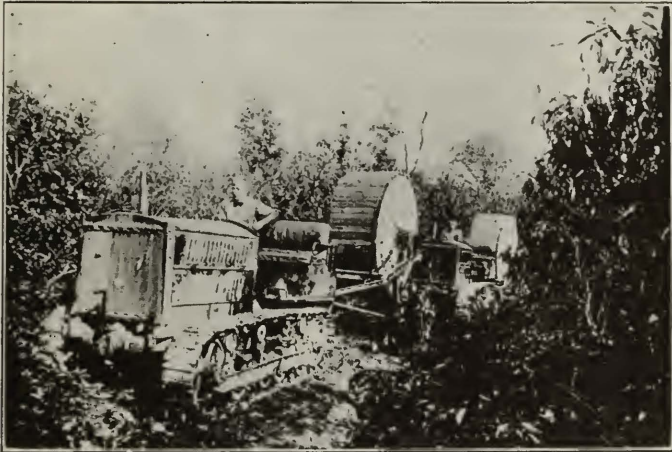
Fig. 12—Tractors Placing Cable Reels in Rough Country
