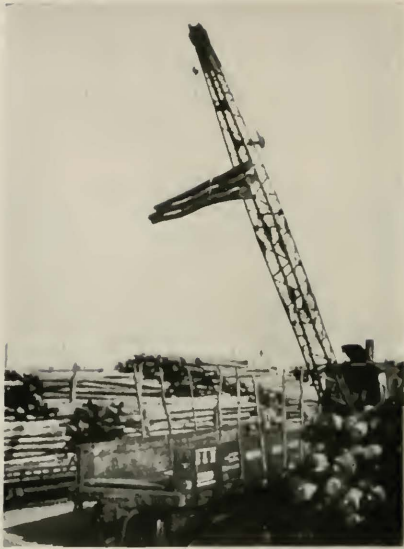
Fig. 17—Handling Poles by Balanced Method with Locomotive Crane
