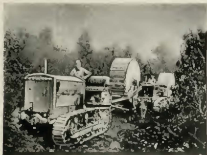
Fig. 3—Transporting cable reels through Allegheny Mountains
