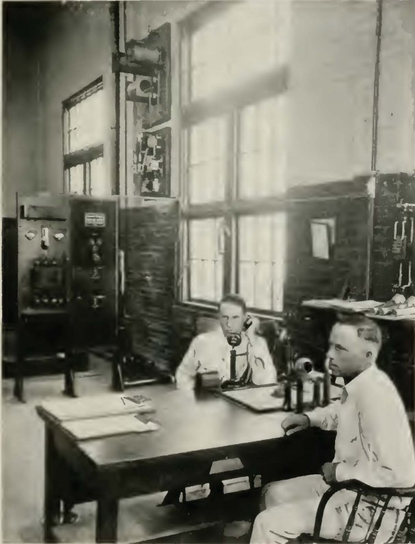
Fig. 26—Typical Power Line Carrier Telephone Installation
