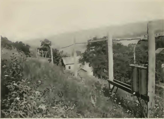
Fig. 9 Toll cable line through open country
