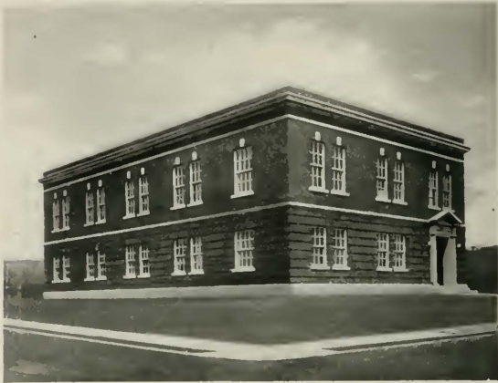
Fig. 5—Typical telephone repeater station
