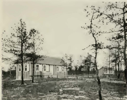
Fig. 2—Exterior of Riverhead Radio Receiving Station
