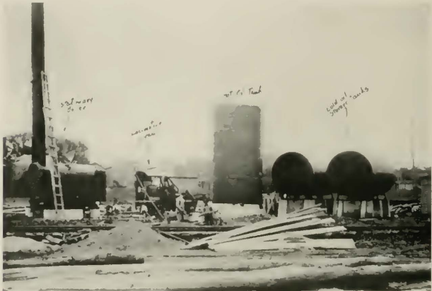
Fig. 30—Steam Boiler During Installation
