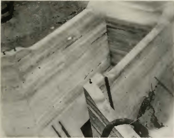
Fig. 25—Concrete Foundation and Protecting Walls for Treating Tanks
