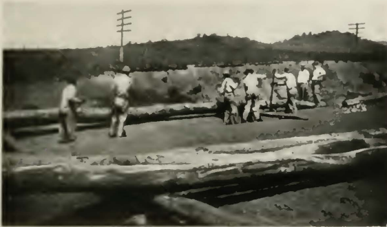
Fig. 13 Handling Poles by Man Power
