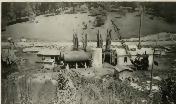
Fig. 22—View of Treating Equipment at Sylva Plant
