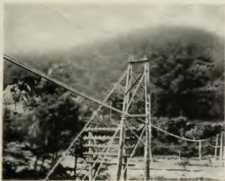
Fig. 4—Toll cable line in Allegheny Mountains
