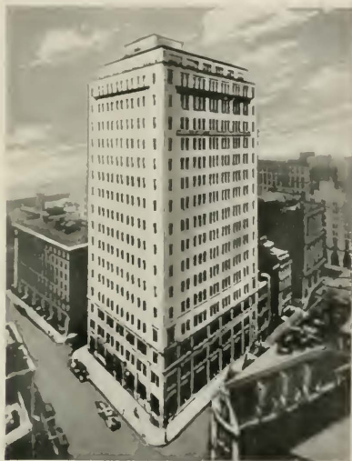
Fig. 15 Bowling Green telephone building, New York City
