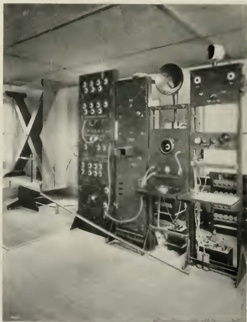
Fig. 3—Interior Riverhead Station
