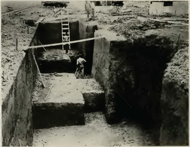
Fig. 24—Excavation for Treating Tanks
