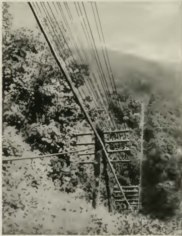
Fig. 10 Cable and open wire toll line in Allegheny Mountains
