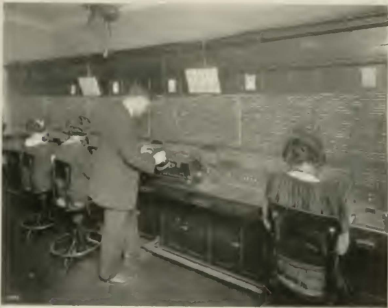
Fig. 7—Illustration of a 3-A Transmission Measuring Set Being Operated in a Manual Office
