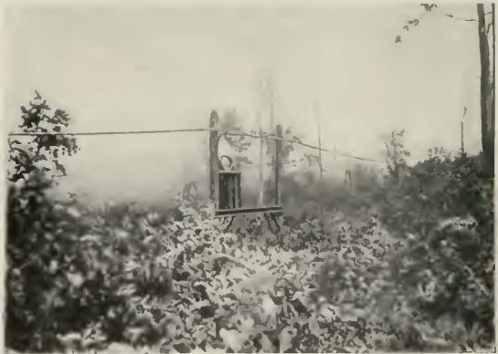
Fig. 8 Toll cable line showing loading coil case
