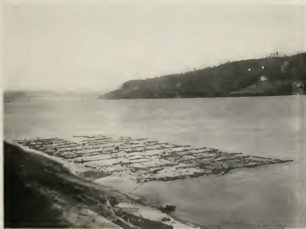
Fig. 10—Four Rafts of Poles at Ceredo Plant
