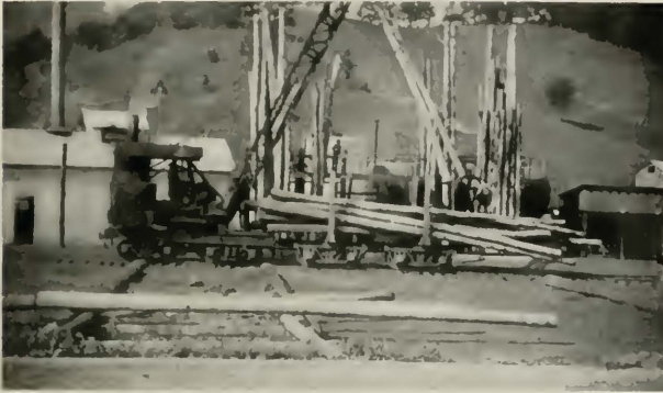
Fig. 16—Unloading Poles from the Treating Tanks to the Dollies, with Locomotive Crane
