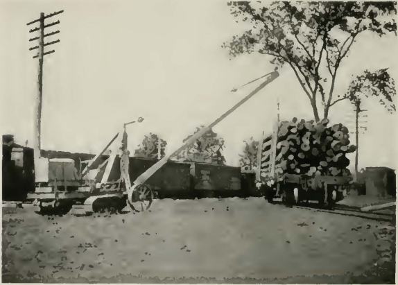
Fig. 8—Car Load of Poles Arriving at the Danbury Treating Plant
