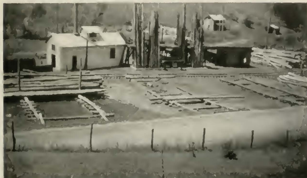
Fig. 19—Preparation Skids Opposite Treating Tanks at Sylva Plant
