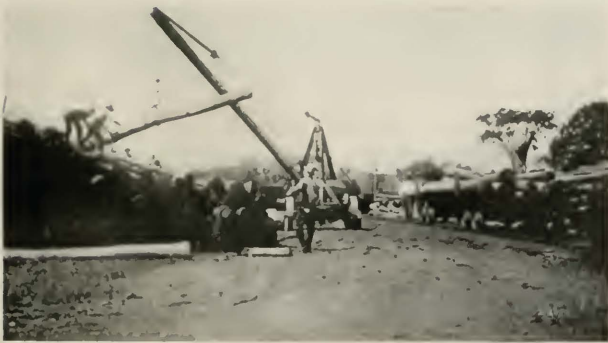
Fig. 14 Tractor Crane Handling Poles from Rail Dollies in Danbury Yard
