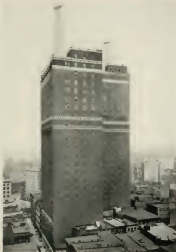
Fig. 17—Long distance telephone building, New York City
