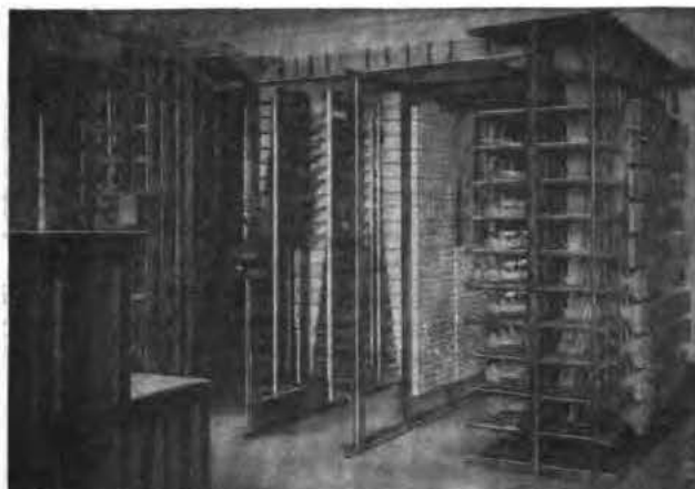
Terminal and Relay Rack.
