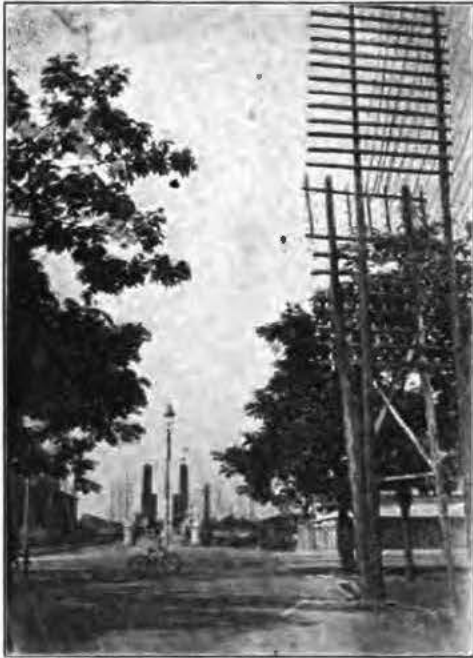
METHOD OF INSTALLING CROSS ARMS
