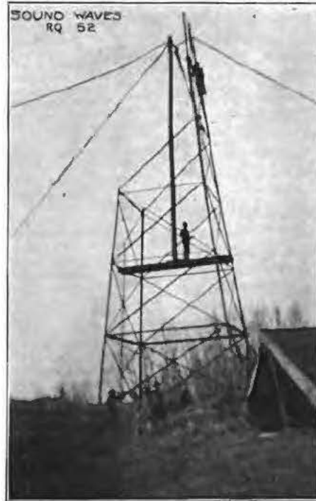
Tower in Course of Construction.
