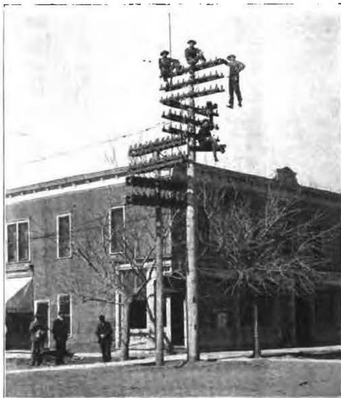
The New and the Old Junction Poles at Elm Creek.
