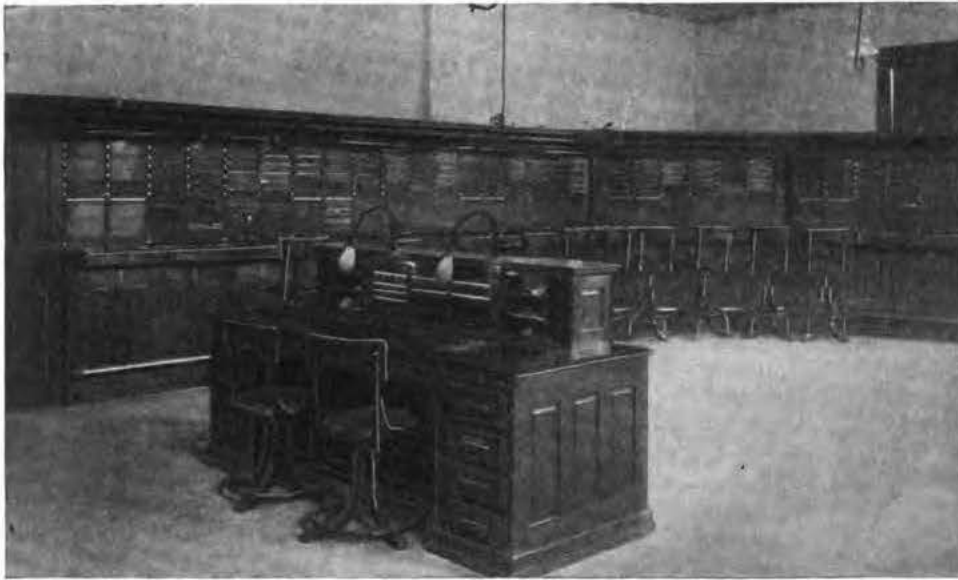
Main Switchboard—Capacity Three Thousand Six Hundred Lines.
