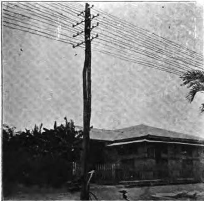
TWO POLES ARE STRONGER THAN ONE
