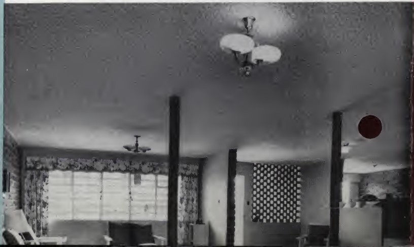
Acoustical Ceiling in Residence
