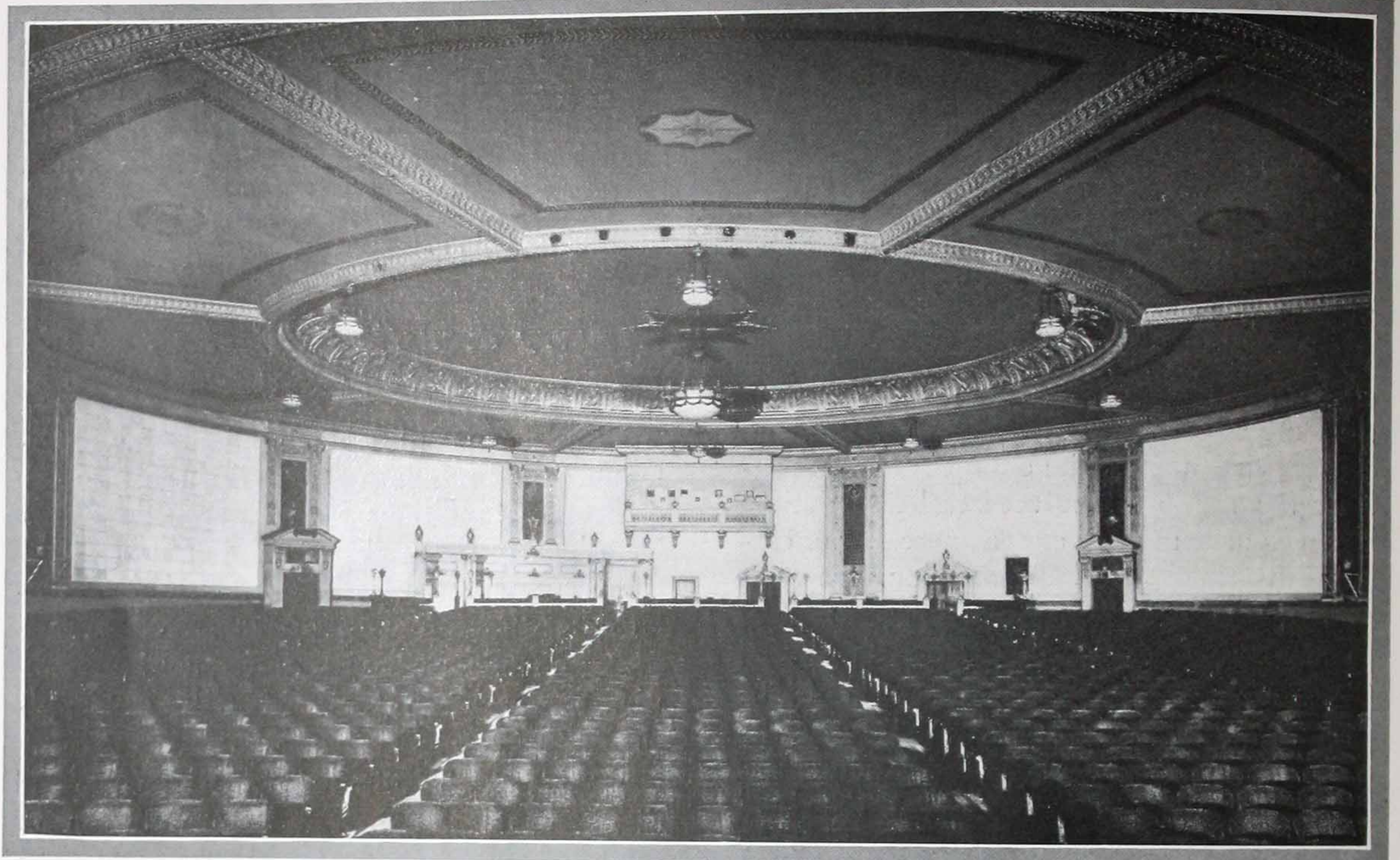
From the above photograph you can get an idea of the size of the Howard Theatre. Note how the panels of J-M Sanacoustic Tile were applied to the walls to correct the faulty acoustics in this auditorium
