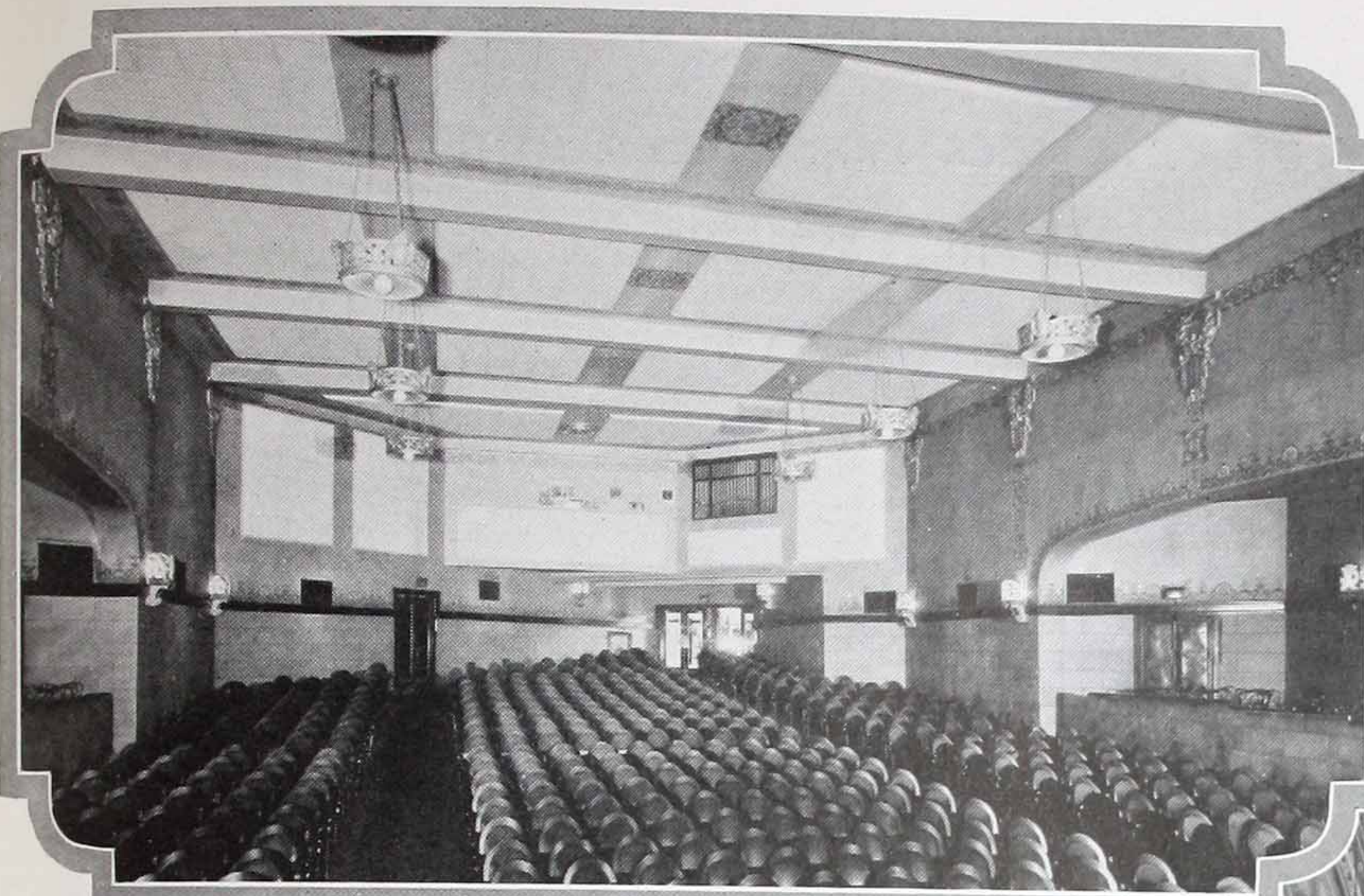
(Left) ANOTHER THEATRE where J-M Sanacoustic Tile was used — the Plaisance Theatre in Chicago, Illinois. Note how the treatment on the ceiling and upper rear wall blends with the tile effect used as wainscoting
